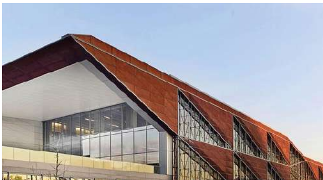
Kasso Cor-ten Steel Façade Cladding
