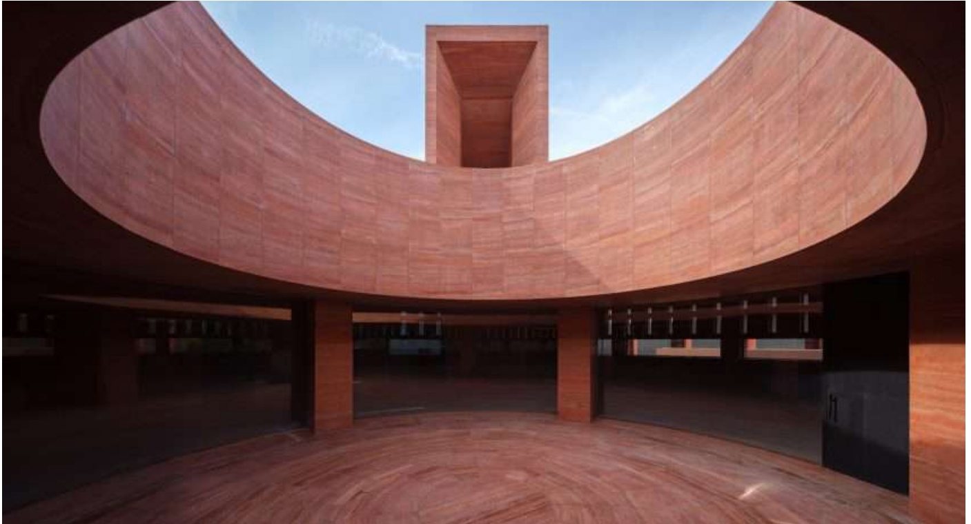
A lightwell connects all floors of the new extension
