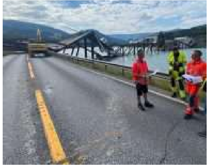
Norway to inspect timber bridges after 10-year-old glulam ...
