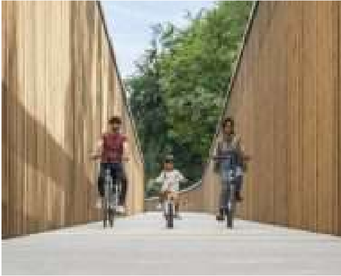
Timber bridge offers visitors 360-degree views of Belgian ...
