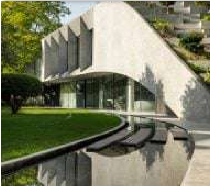
Villa KD45 is a concrete house in Delhi with a plant-covered ...
