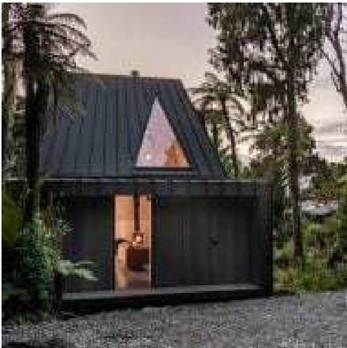
Fabric builds CLT vacation cabin in New Zealand rainforest
