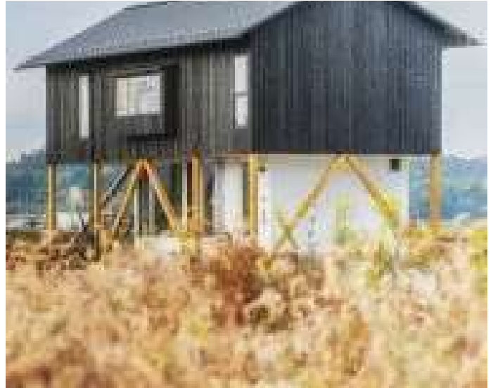
Ushijima Architects designs flood-resilient U-House near Japanese lake
