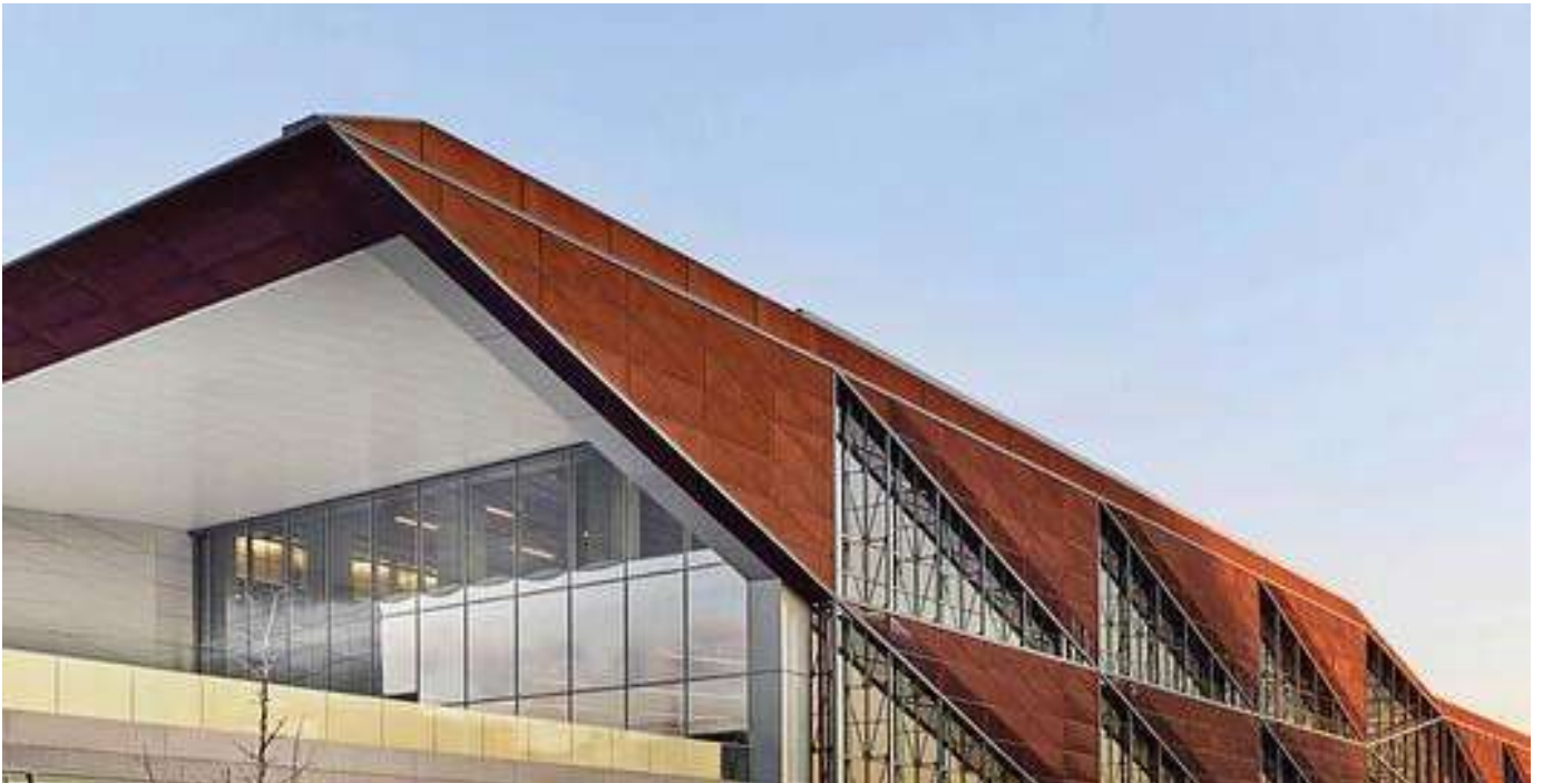
Kasso Cor-ten Steel Façade Cladding
