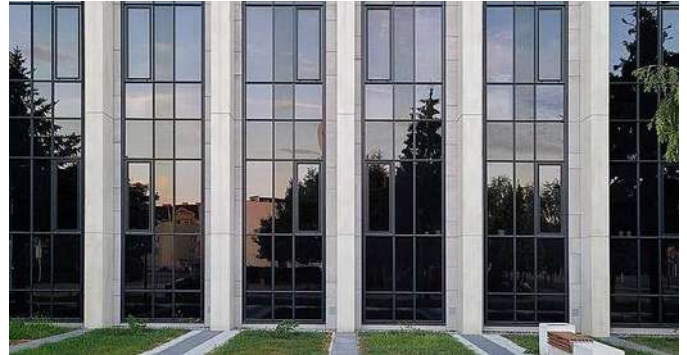
Grespania Coverlam Wall Cladding on University Facade
