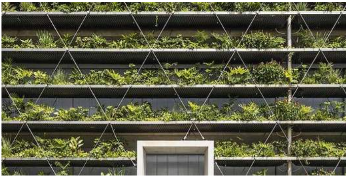
Jakob Green Walls in Jakob Saigon Factory
