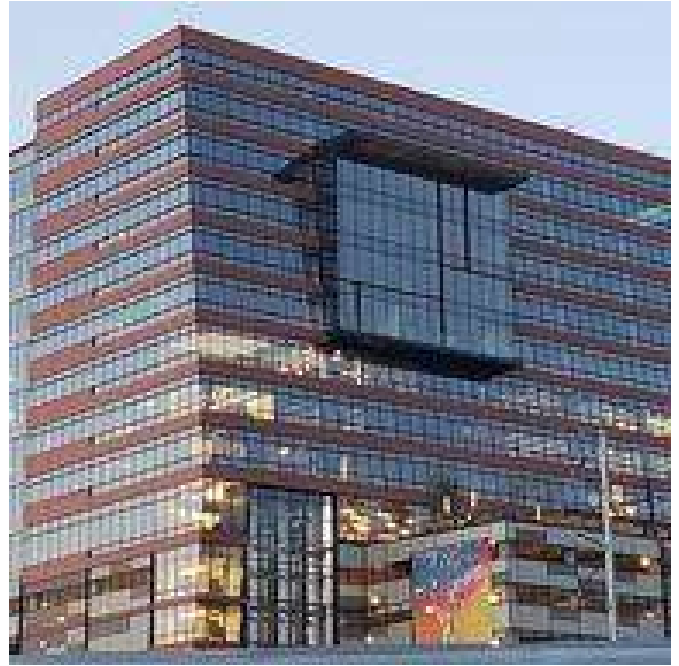
Morin Corp. Metal Cladding in The Dillon
