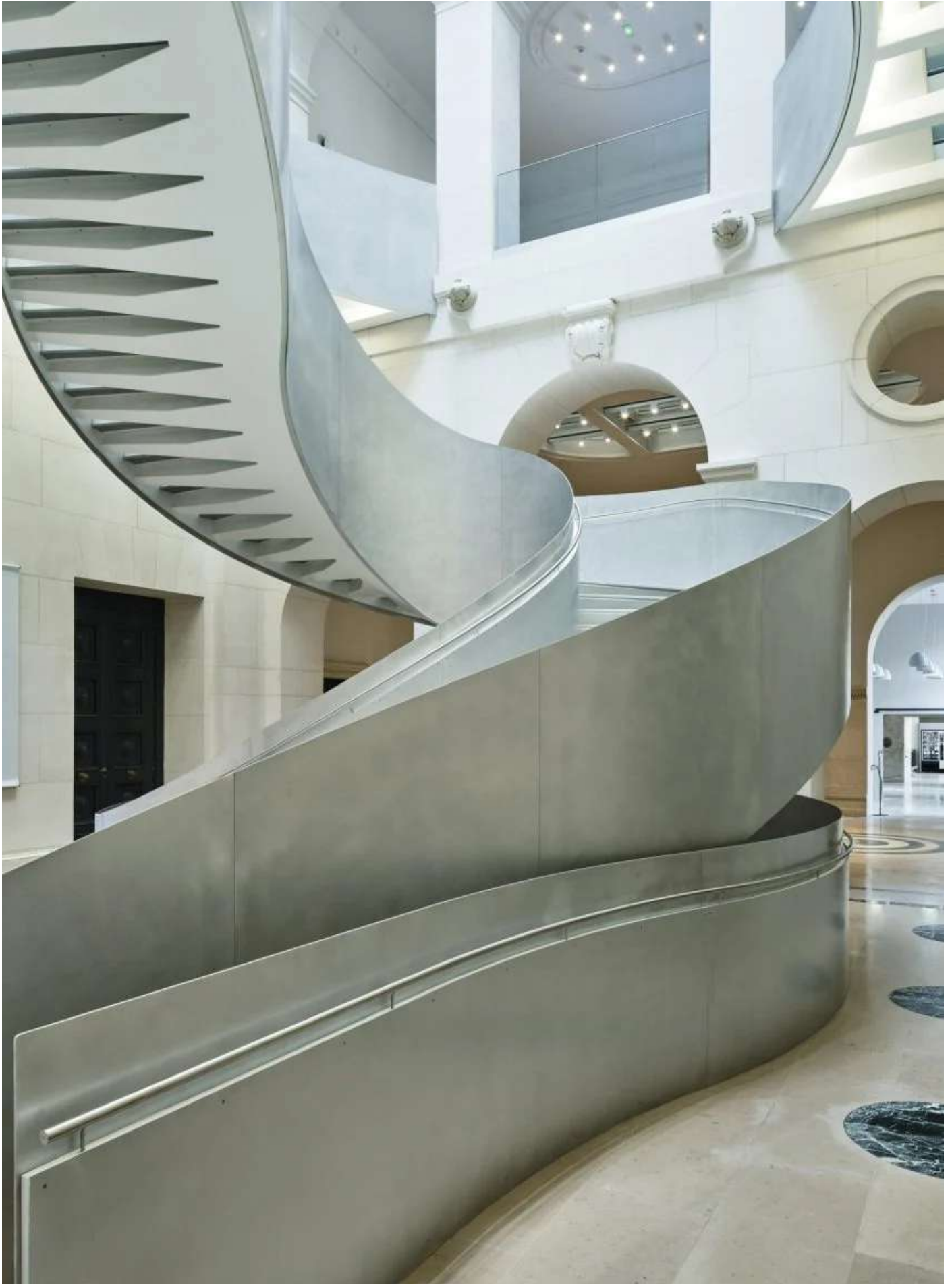
An aluminium-clad spiral stair has been introduced
