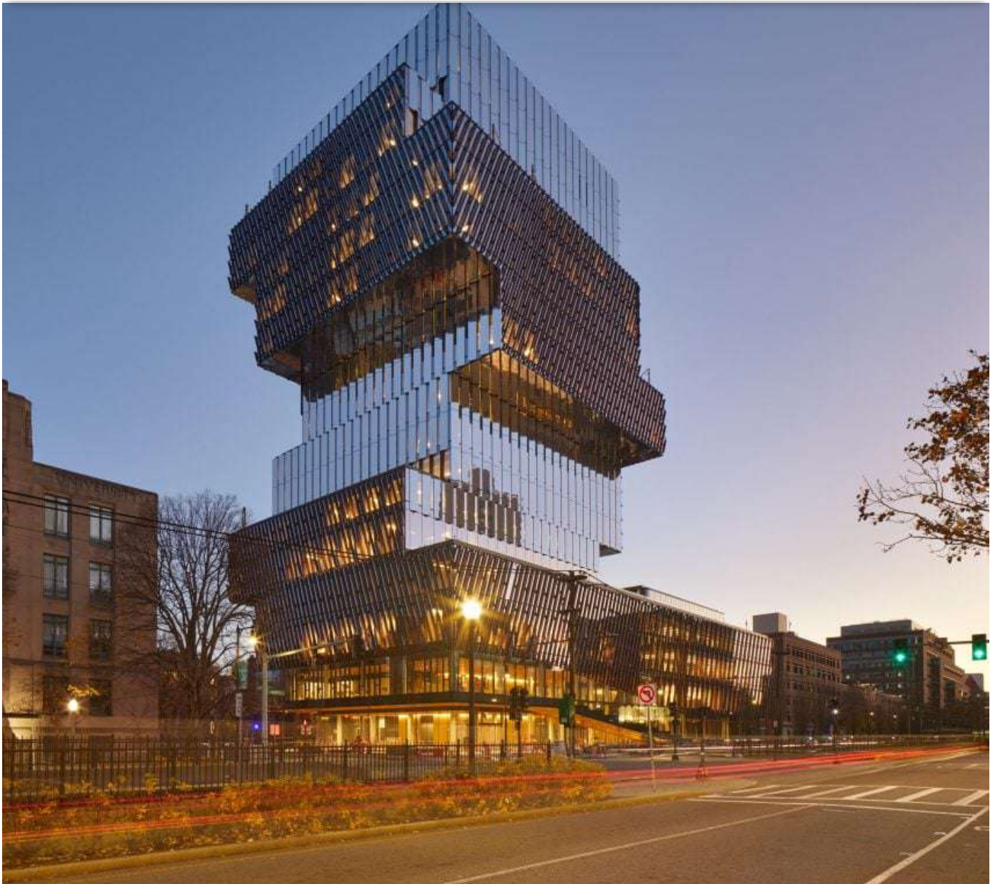
The facade has a series of diagonal louvers
