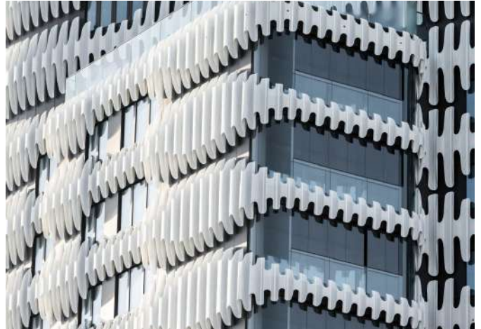
J Mayer H wraps RKM 740 Tower in wavy metal cladding
