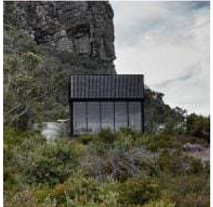
Steel and timber cladding helps remote hiking shelters blend in with Australian landscapes
