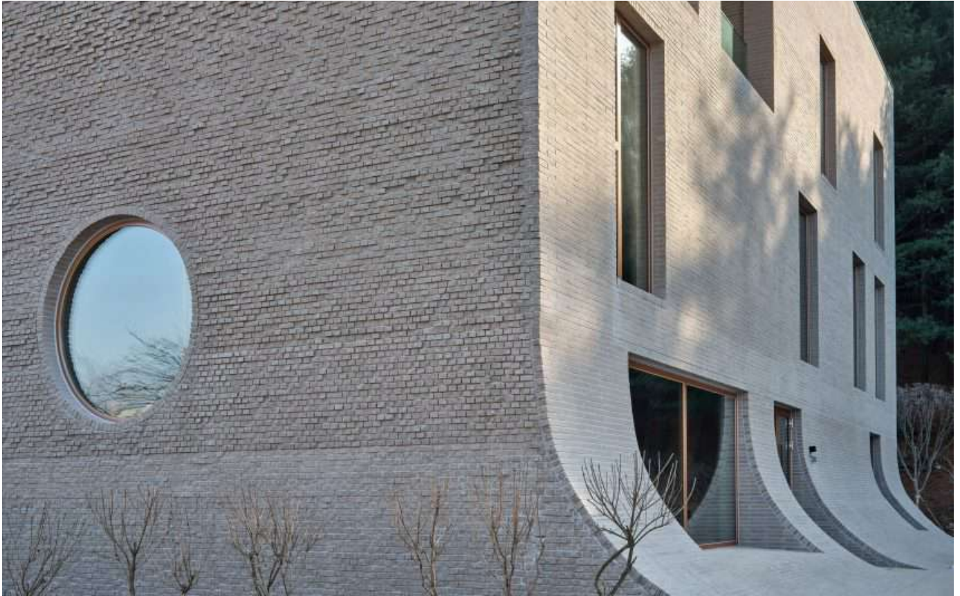
Concrete brick walls slope down into the floor of the courtyard at Café Teri
