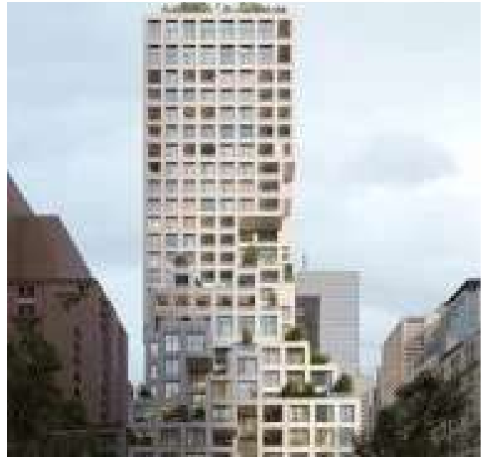
ODA's "fractal" skyscraper latest addition to Billionaire's Row
