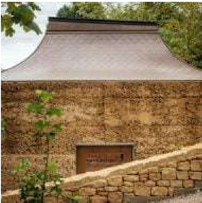
Invisible Studio adds rammed-earth yoga studio to the gardens of Somerset hotel
