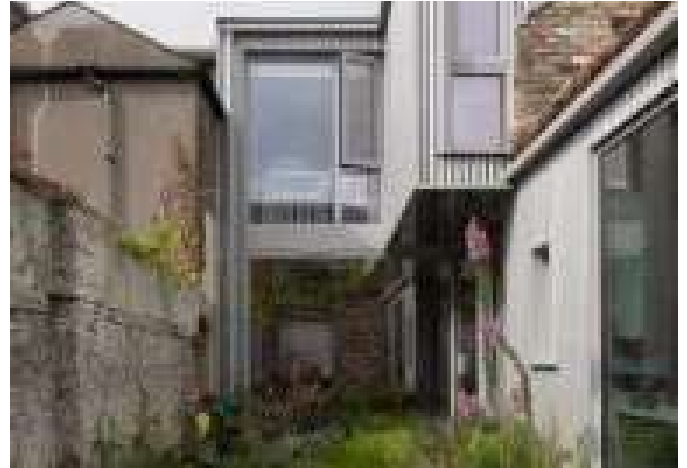
Scullion Architects adds corrugated metal-clad extension to Dublin cottage
