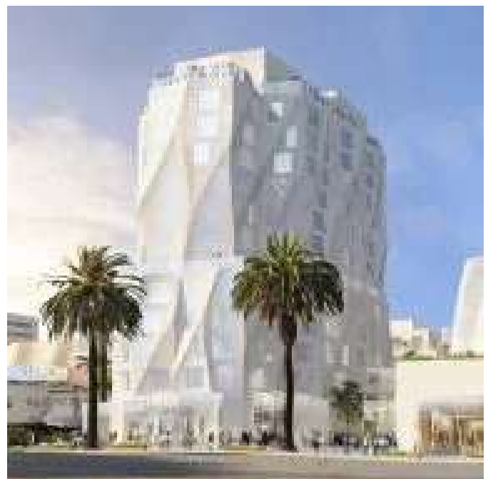
Frank Gehry's long-awaited Ocean Avenue Project gets final go-ahead in California
