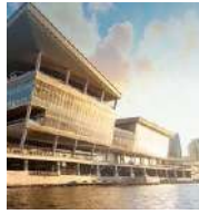
Kryton Concrete Hardening – Har...
