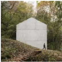
Carvalho Araújo completes monolithic concrete house in a Portuguese forest
