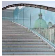
Venice to replace glass tiles on Santiago Calatrava-designed bridge amid "almost daily" falls
