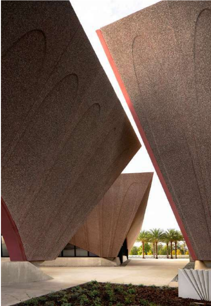
The three structures were constructed using pigmented concrete
