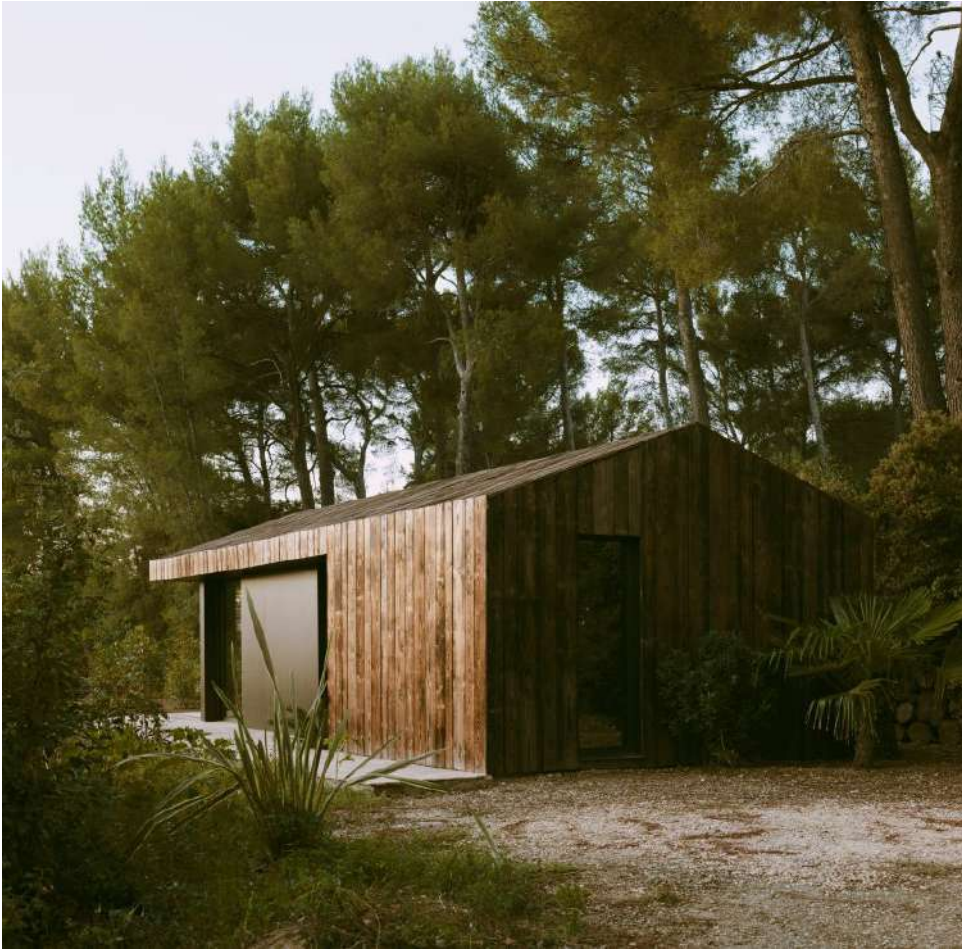
It is clad in planks of scorched wood
