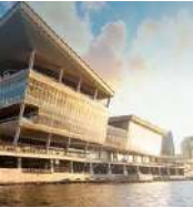
Kryton Concrete Hardening - Har...
