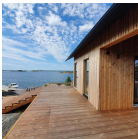
Lunawood Thermowood Façade and Decking in Project Ö|Lunawood
