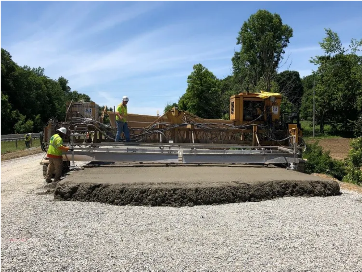
Sensors installed on Indiana interstate I-74. Erin Easterling/Purdue University, CC BY-ND
