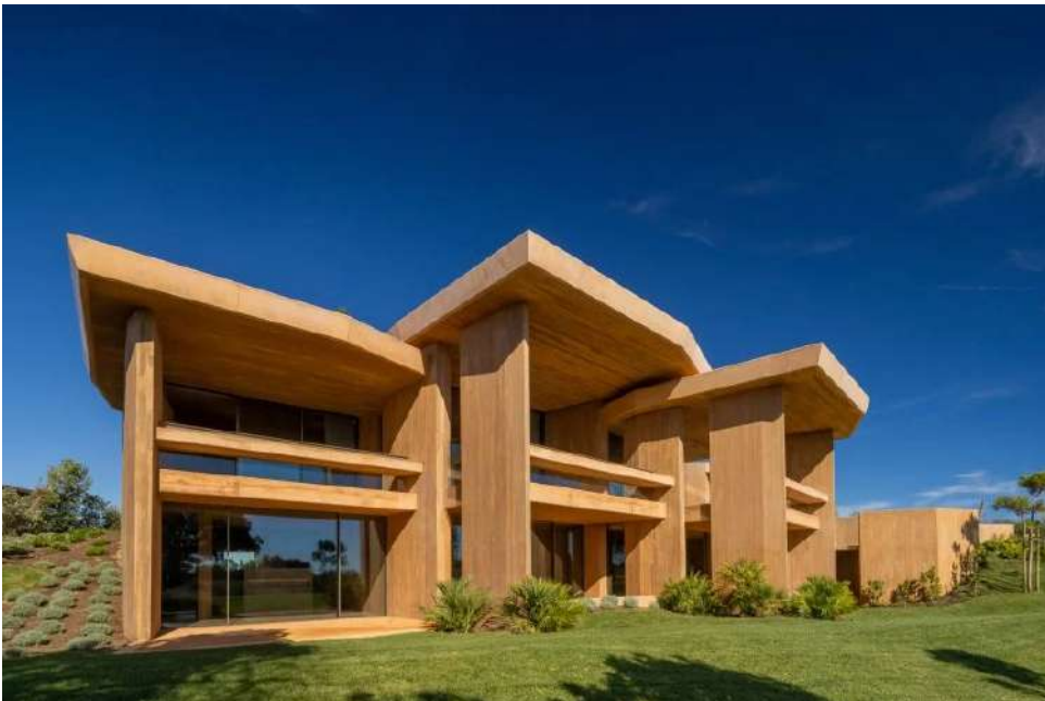
Overhanging roofs offer natural sun shading
