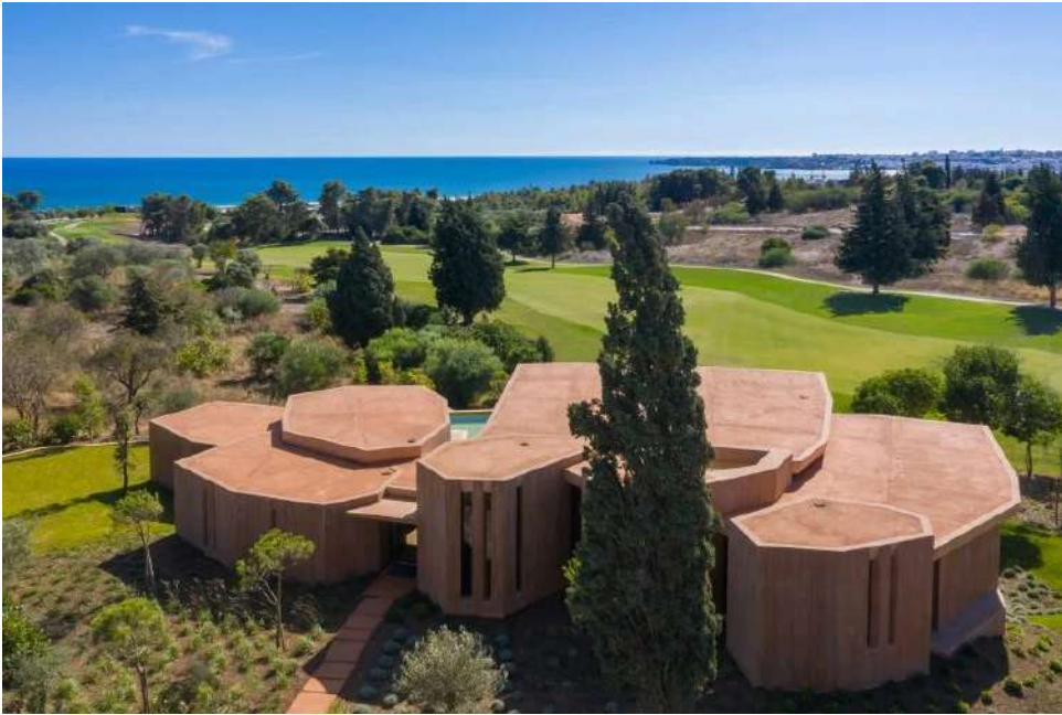
The building is constructed from red pigmented concrete
