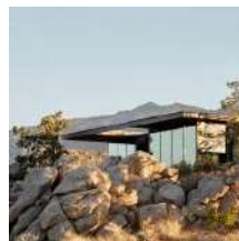
Boulders and pine trees surround High Desert Retreat by Aidlin Darling Design
