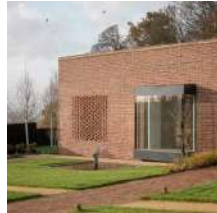
Only one of 20 RIBA House of the Year longlisted projects achieved top sustainability grade
